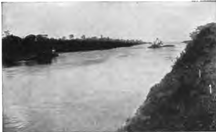
Mindi Excavation, Looking North from East Bank of Canal
